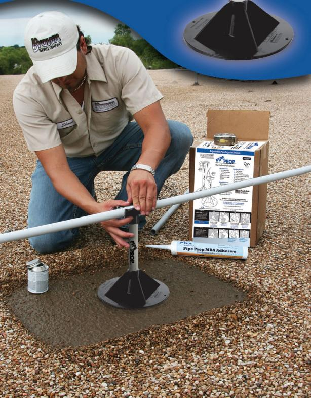
**Pipe Prop Is an Adjustable Pipe Support System that Elevates and Secures Industrial Piping on Commercial Roofs**
